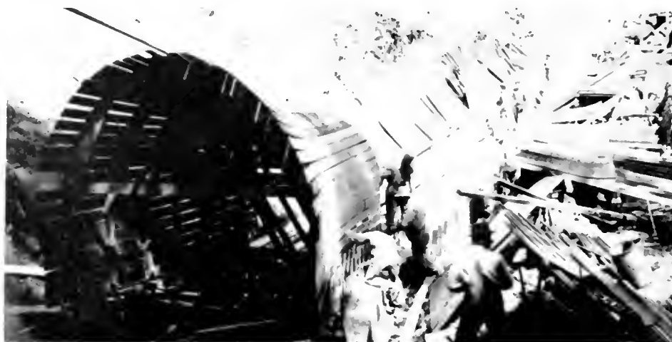
FIG. 20. Forms for throated entrance to concrete arch culvert. Note gradual flattening of grade towards outlet
